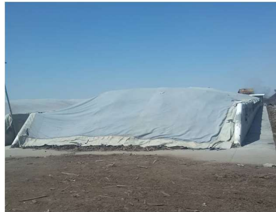
Covering the heap with membrane
